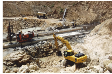
Middle plinth improvement
