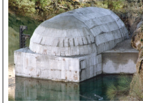
Submerged intake structure
