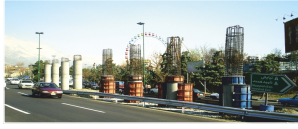
Construction of bridge pier and head in heavy traffic
